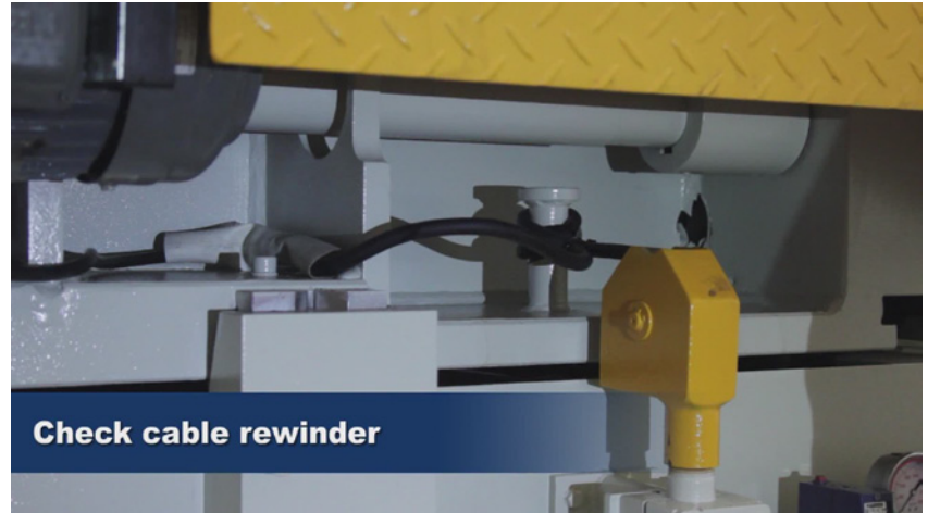
Check cable rewinder
