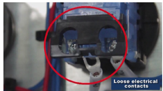
Checking electric point
