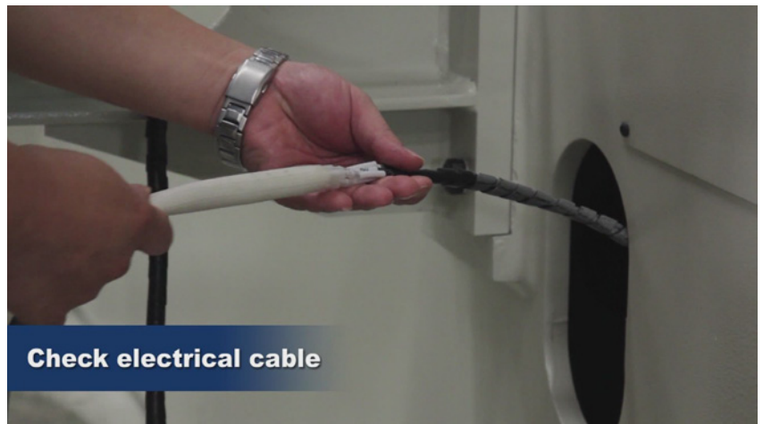
Check electrical cable
