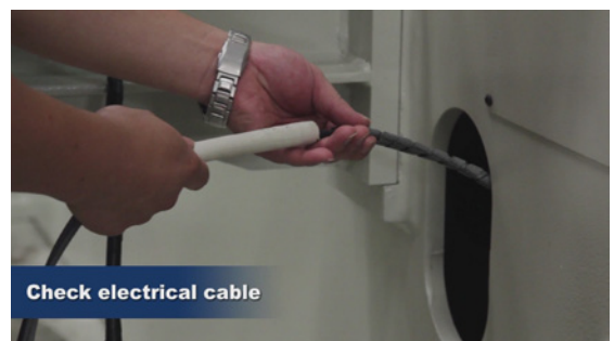
Check electrical cable
